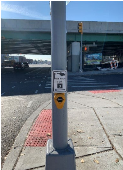
Figure 74: ADA-compliant ramps and pedestrian push button, Intersection of Bronx River Ave and Bruncker Blvd
