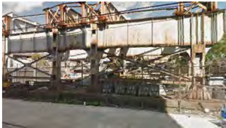
Elevated structure of the former 180th Street -Bronx Park Station on Lebanon Street (2014).
